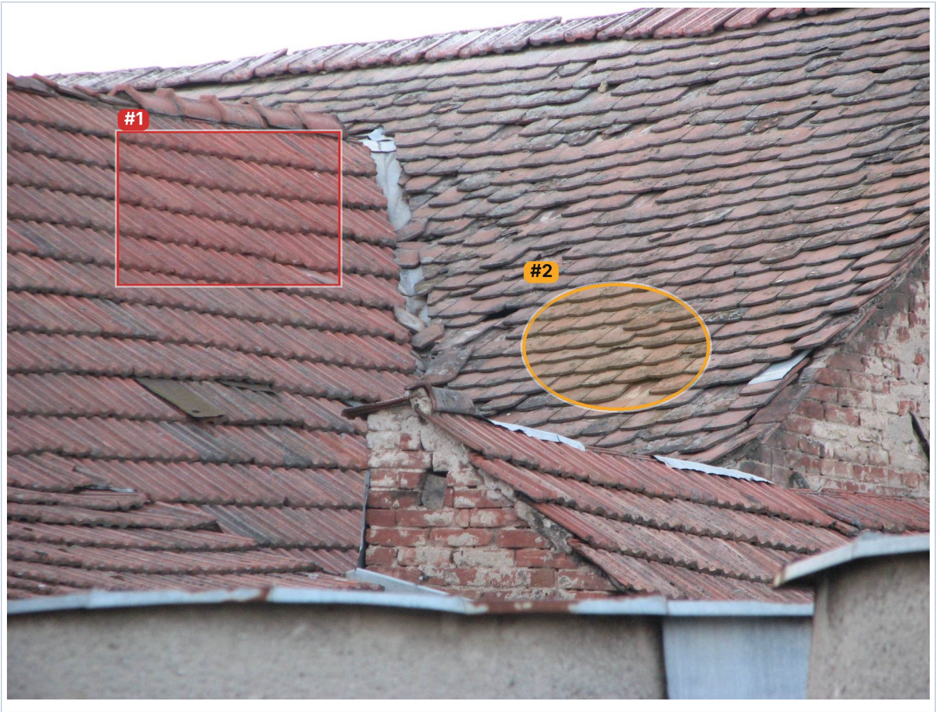
Photograph 1 — Ridge capping at gridline 7 (Main roof)
