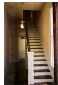
Plasterboard joint showing through the paint
