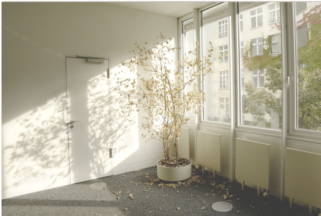
Kitchenette with removed units
