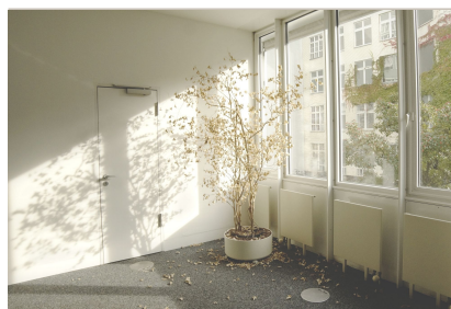
Damaged partition at the former meeting room
