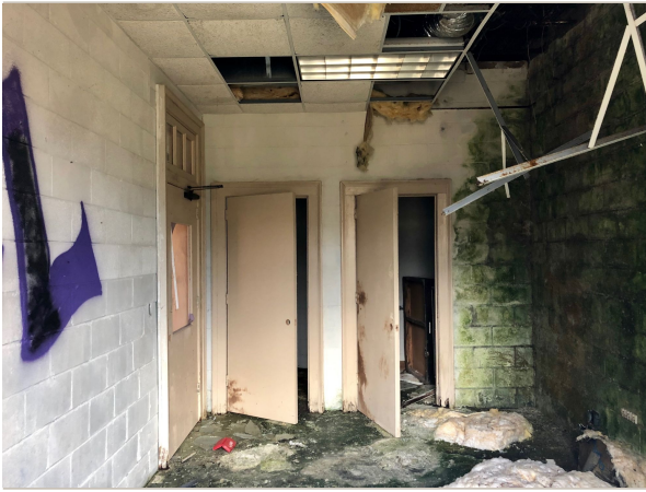
Kitchenette with removed units
