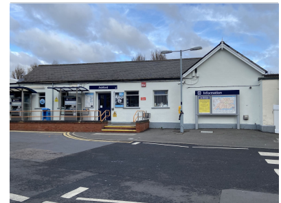
Principal entrance ramp and steps
