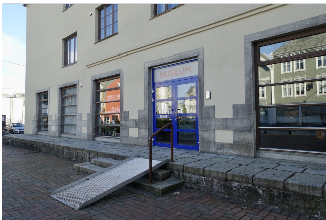
Principal entrance ramp and steps
