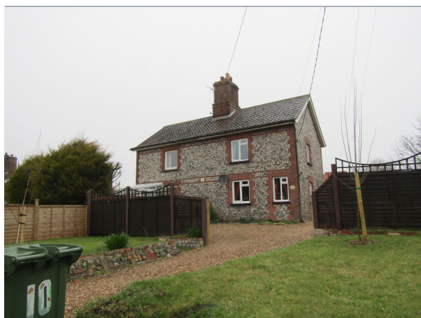
Roof covering from the garden
